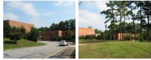
Exterior Photos - Music Building
