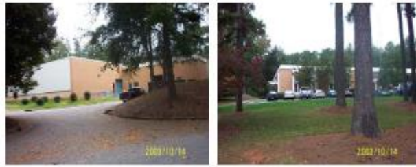
Exterior Photos - Maintenance Building
