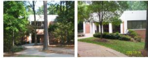
Exterior Photos - Technology Building
