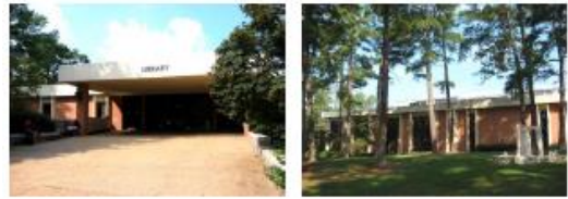
Exterior Photos – Library Building
